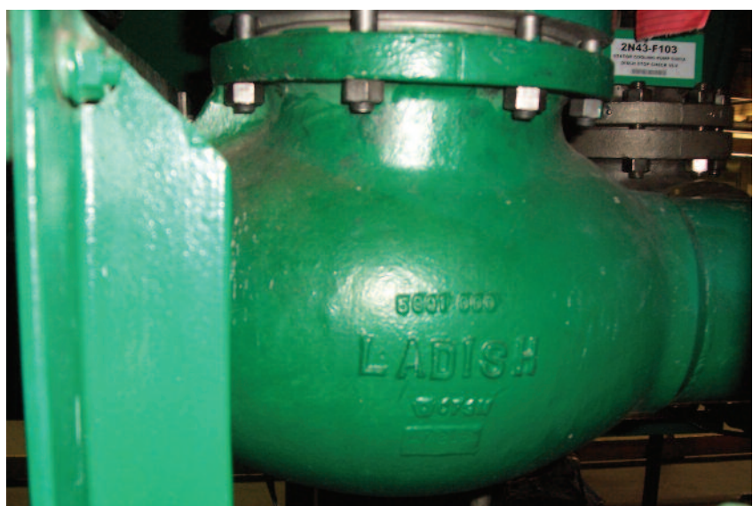
Counterfeit (top) and legitimate (bottom) valves at a southeast US nuclear power plant. One counterfeit valve had been installed in a non-safety application; a second was in inventory.
